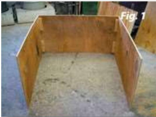
1. Attach 2 pieces of 2x2x6" block to side panels. Position them flush with the edge, allowing 1 1/2" top & bottom clearance to allow for more block placement. (See Fig. 1)
